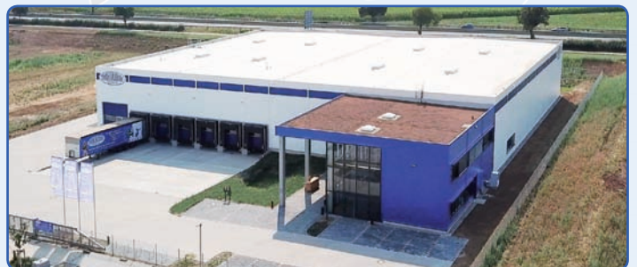
Logistics and training center in Bensheim
